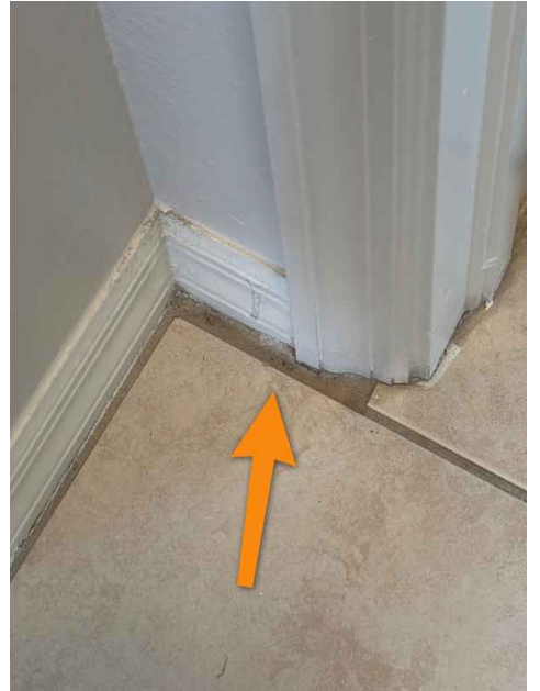
Hallway to guest bedroom, NW
